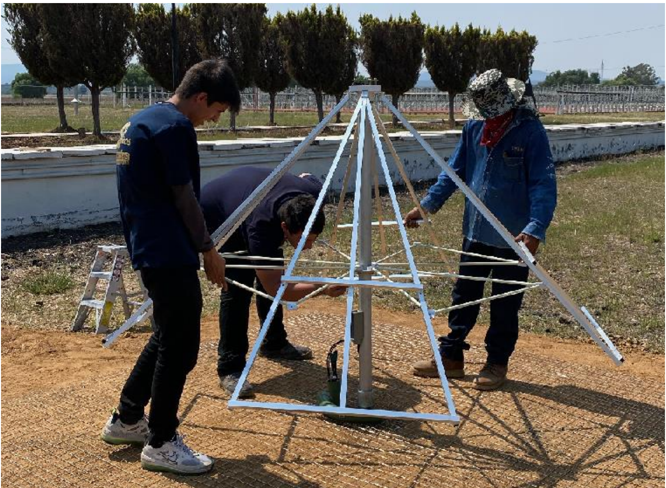
Fig. 3: Installation of LWA in Mexico. (From left to right: Marco Medina-del-Angel (student); Oscar Godines-Torres (student); Ernesto Andrade-Mascote (head of technical staff at MEXART))
