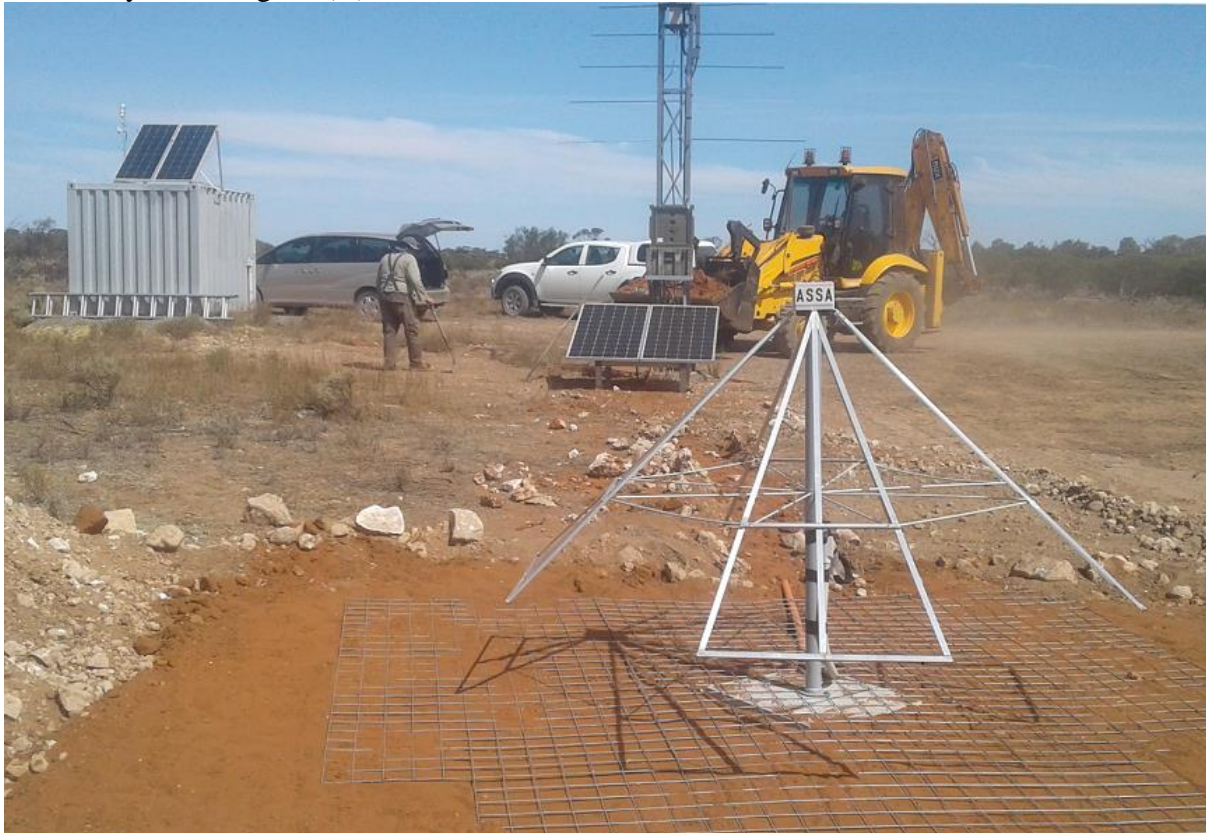
Fig. 3: LWA installation at ASSA, Australia. https://www.assa.org.au/
