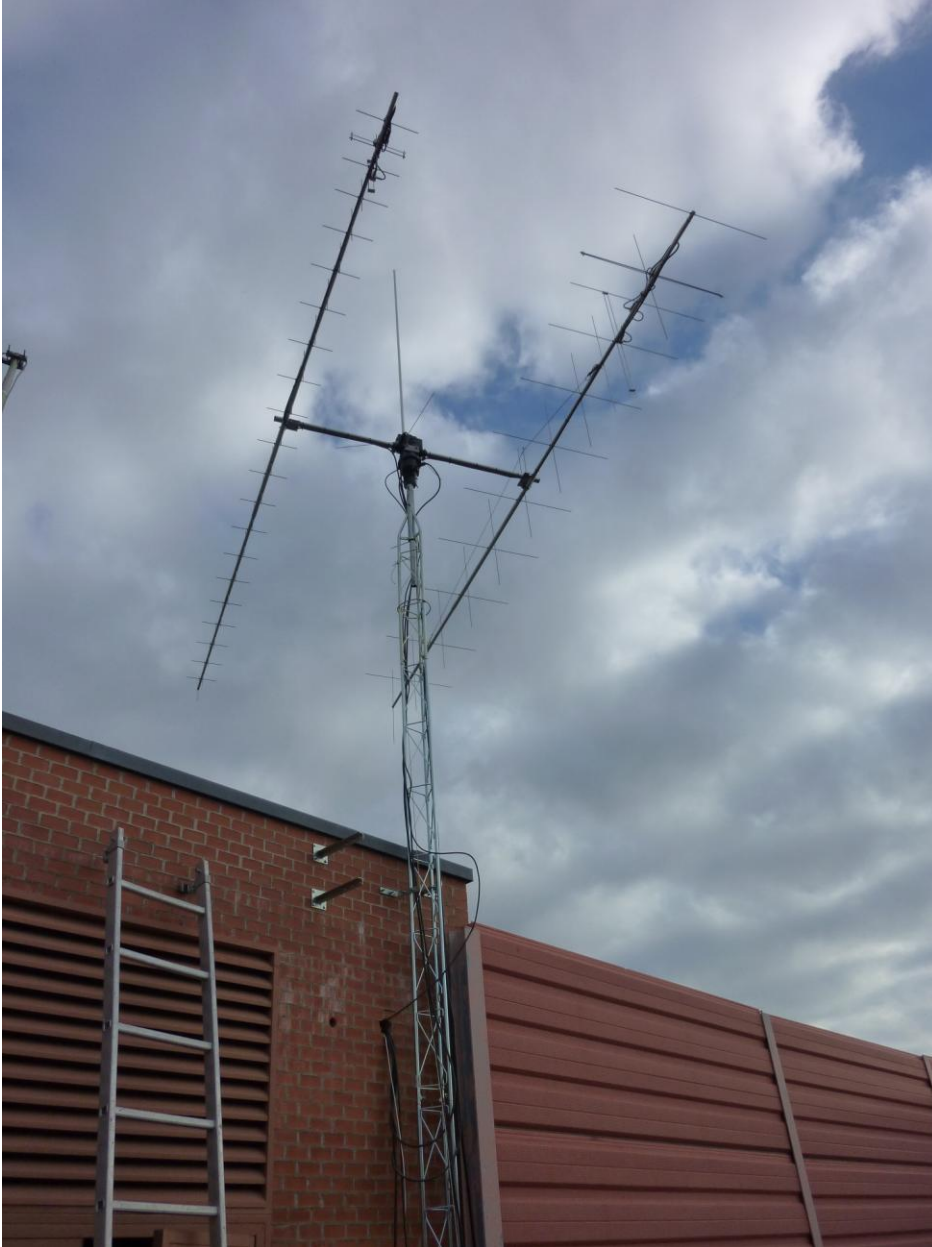
Fig. 4: Yagi antennas on a two axis antenna rotator, tracking the Sun
