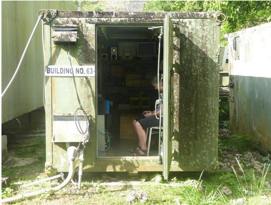
Fig. 17: Full metal shed containing ionosonde and 2 Callisto
