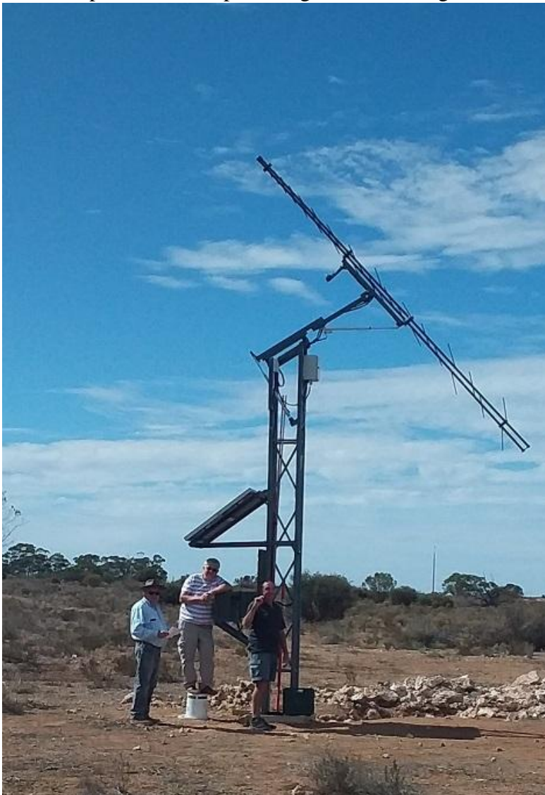
Fig.2: Antenna (LPDA) and mounting at LMRO.
