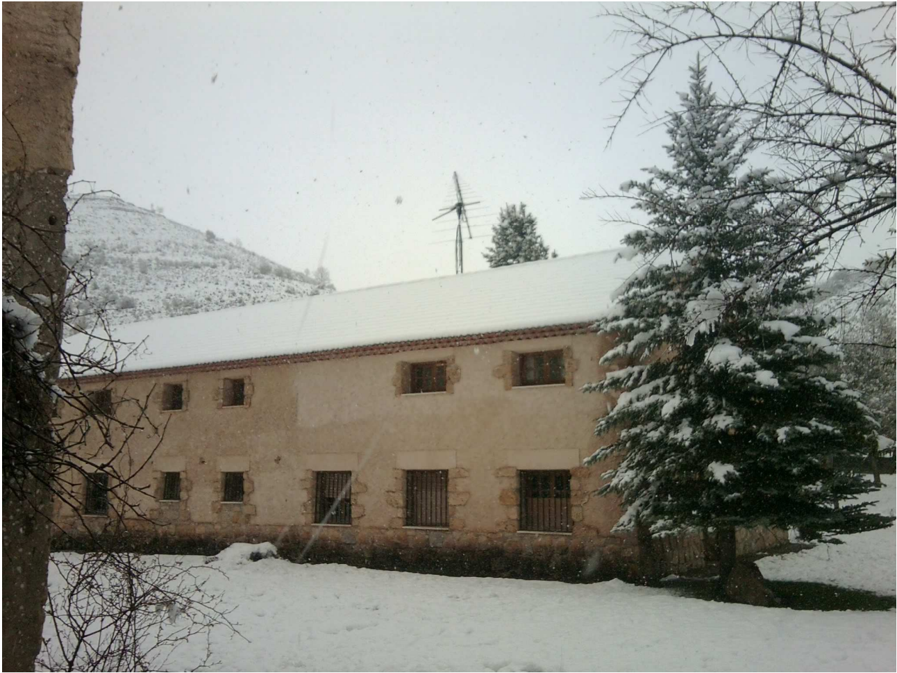
Fig 3: Log-per antenna on top of the roof with tracking system. Photo by Andrés Russu
