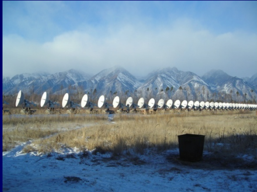
Antenna farm at SSRT
